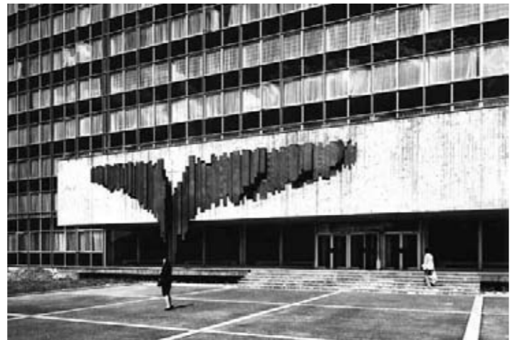
Reliéf po instalaci (archiv Vladislava Gajdy, foto Petr Sikula) / Relief after installation (archive of Vladislav Gajda, photo Petr Sikula)
