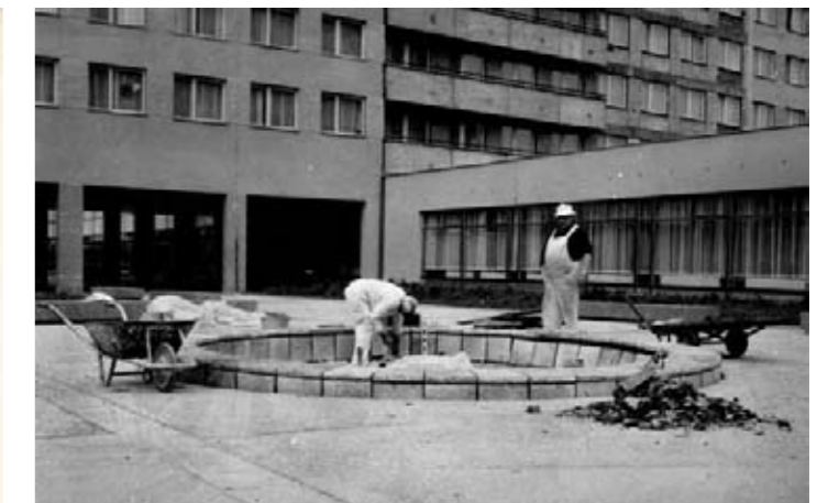
J. Myszak s pomocníkem při pracích na osazení fontány / J. Myszak with his assistant during installation of his fountain
